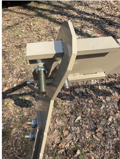
Both retention bolts installed, opposite sides of the joint, same direction.
